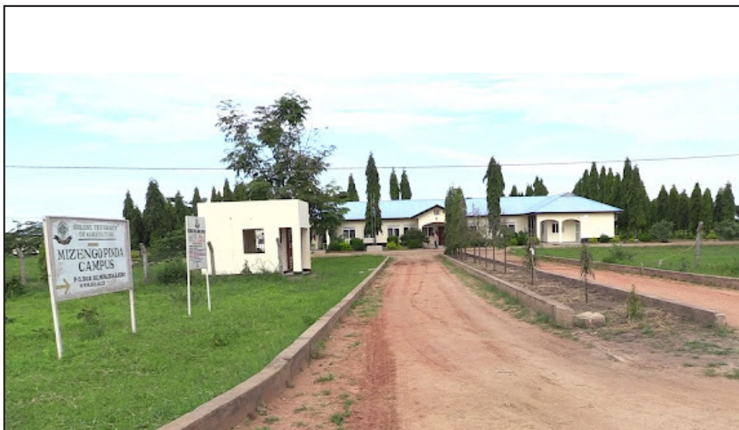
Front view of the Campus Administration building at Mizengo Pinda in Katavi Region
